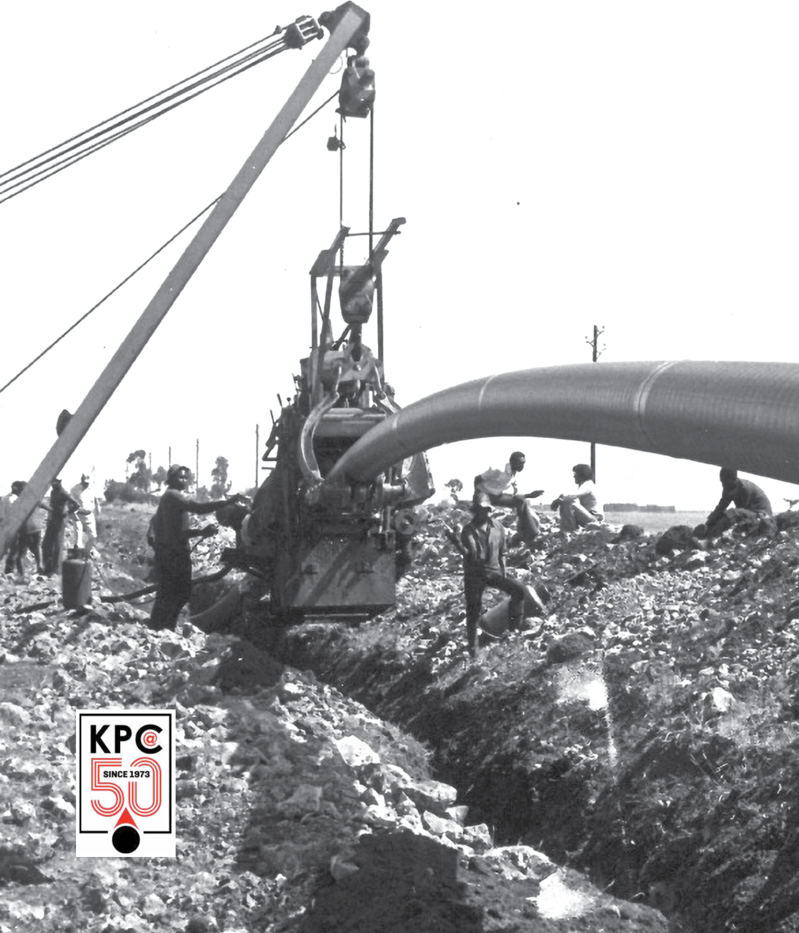
Construction of the Nairobi- Mombasa pipeline.
