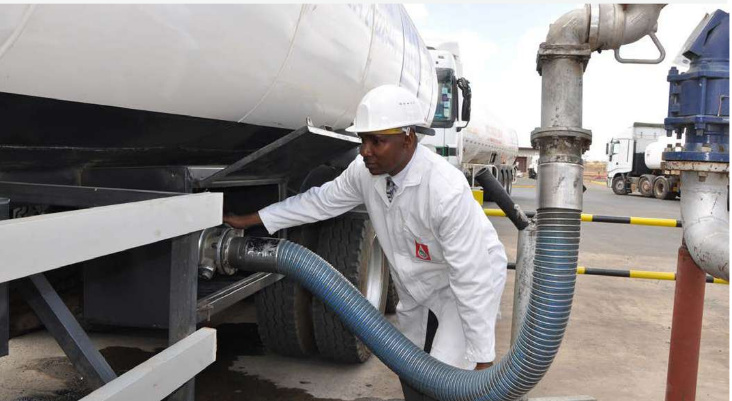
Bottom loading of a truck at Eldoret Depot
