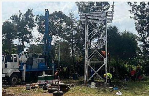
Borehole drilling and equipping at St. Patrick Secondary School in June 2024.
