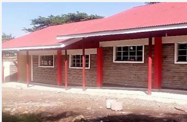
Completed Classrooms at St Joseph Junior Secondary School in March 2024.
