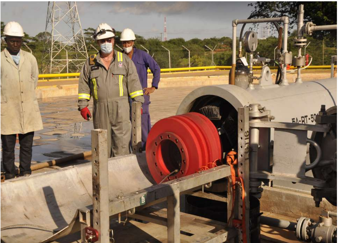
Pipeline inspection (pigging) process at PS 7 to ensure the integrity of the pipeline.
