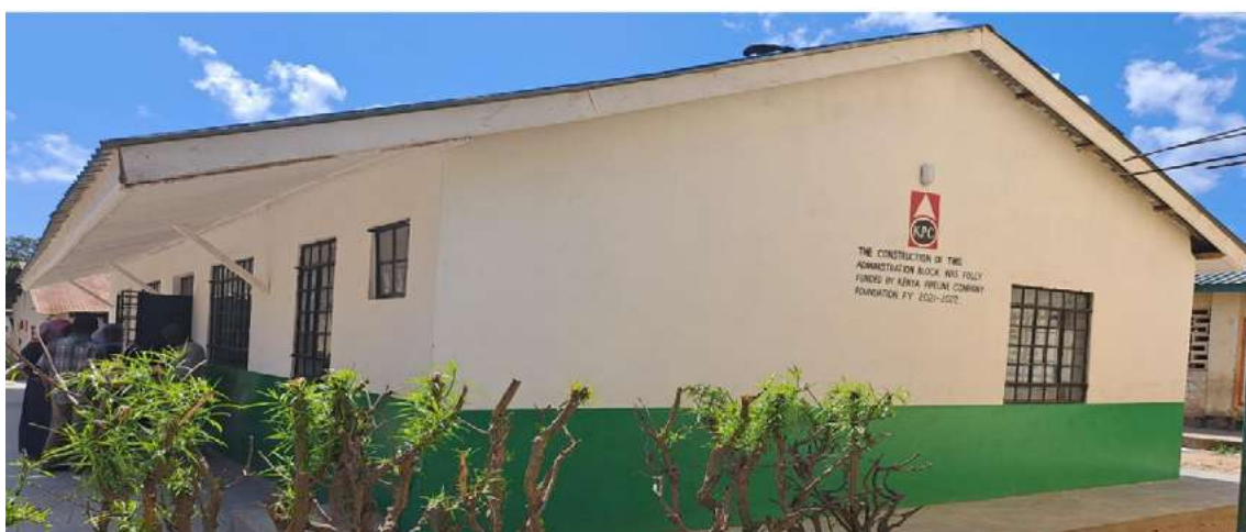
KPC Foundation sponsored the construction of an administration block at a cost of KShs 4 million at Kwahola Primary school in Mombasa County.
