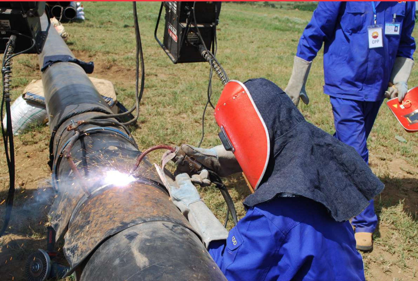
Welding of pipeline
